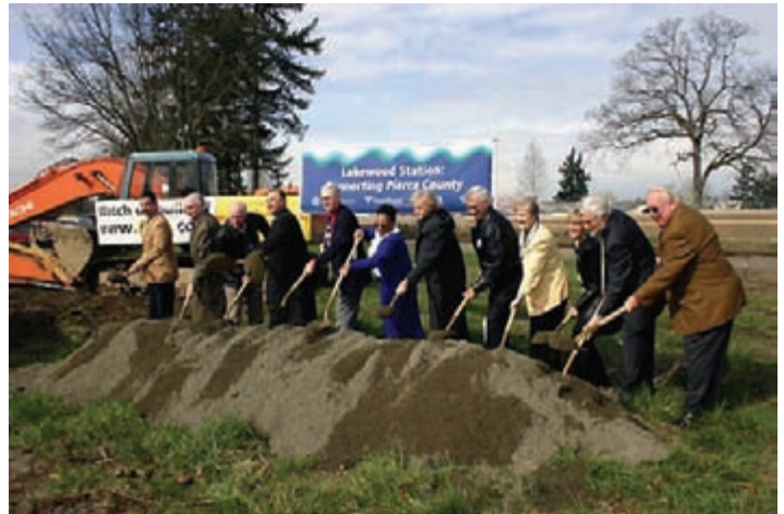
City leaders join other local and regional officials on March 30, 2007 in breaking round at the Lakewood Sound Transit Station that will open in 2008.
