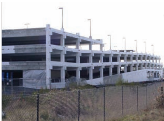
Sound Transit Station—in progress
