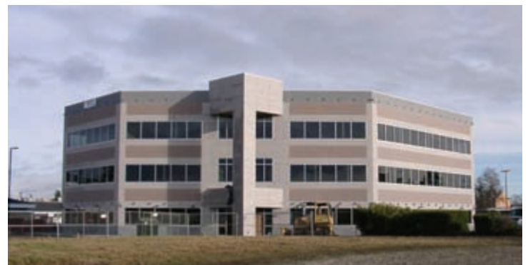
Harborstone Credit Union HQ Building
